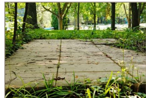
The cement slab can still be seen behind the bench that looks over the lake at the top of the hill, west of the main park. See top of page 9 for picture of original cottage.
